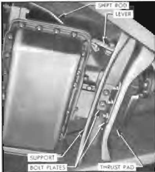
Figure 4-71—Left side of Dynaflo Transmission Installation
